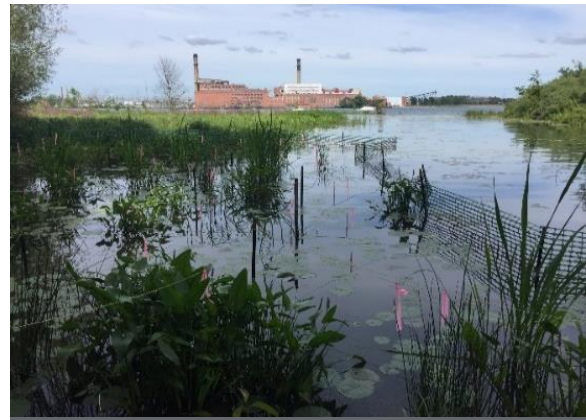
An eroded shoreline at a former ferry slip in Beaver Island State Park was regraded and planted with native riparian species. The inlet now offers sheltered areas for improved fish habitat.
